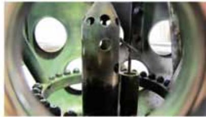
Pilot light and Burner Ring
