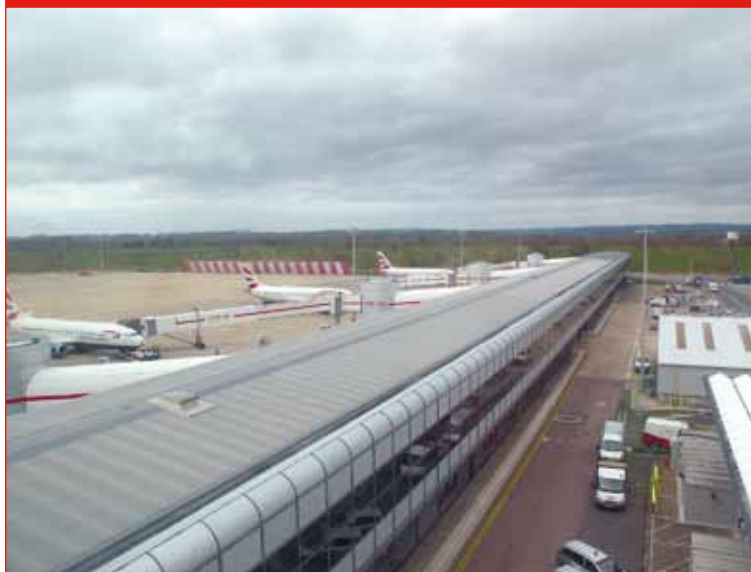
Picture 12: Pier 6 at Gatwick Airport
