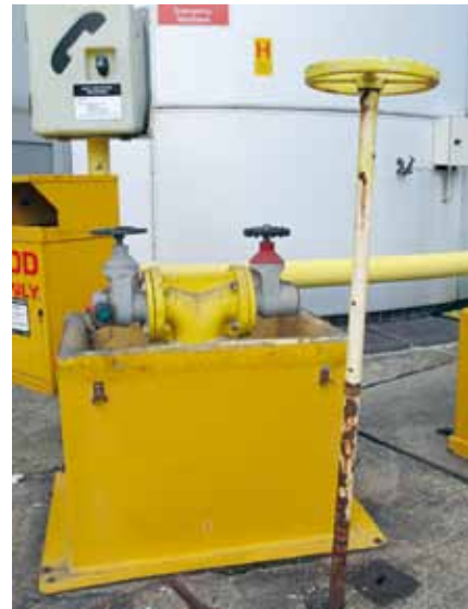
Picture 24 and 25: Pillar hydrant and control valves with insulated boxes
